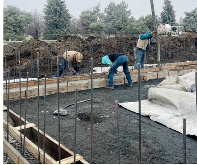
Pouring the new Lewis building footings in December.
