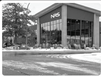
Commercial Glass & Storefront Buildouts
