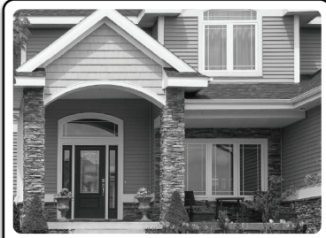
Residential Window & Door Replacement
